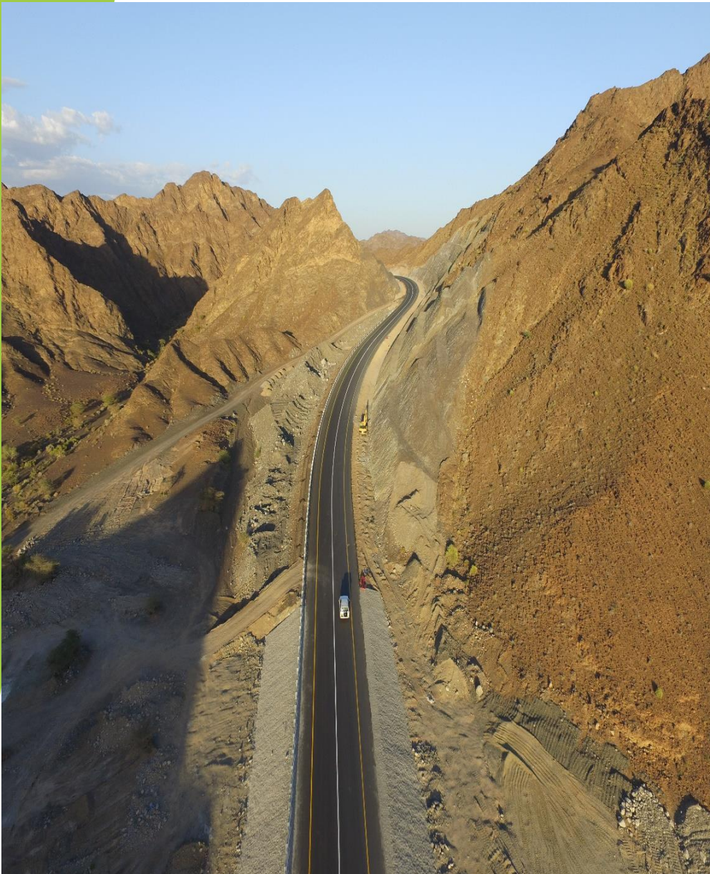
HILL CUTTING BOTH SIDE CH: 7+500
