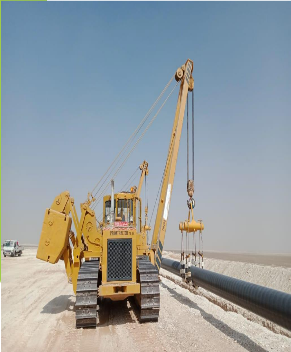
TRENCH EXCAVATION & PIPE LAYING
