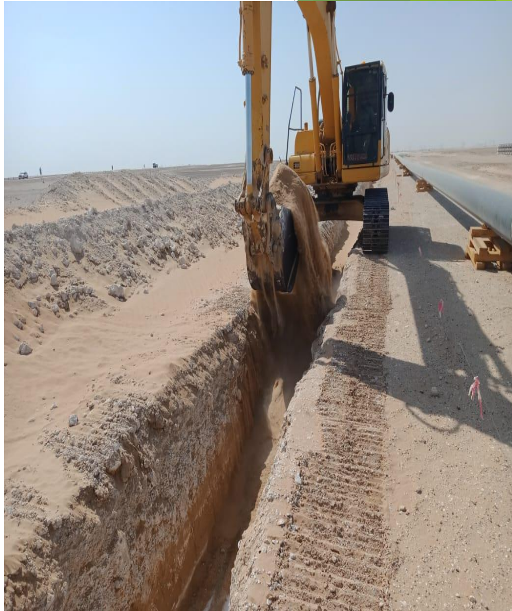
TRENCH EXCAVATION & PIPE LAYING
